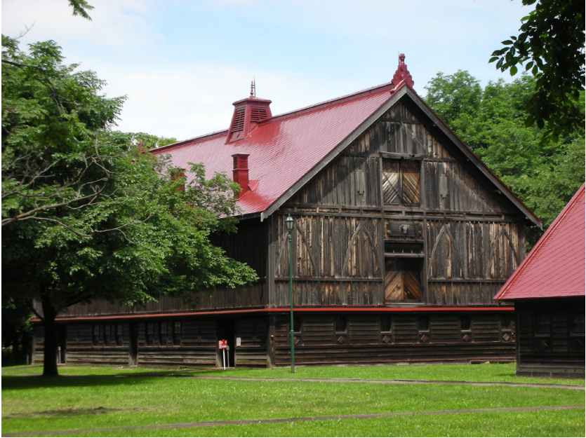
Sapporo Agricultural College Model Dairy Barn, located on the campus of what is now Hokkaido University. Completed in 1877, the barn was inspired by a similar structure at Massachusetts Agricultural College. Photo by author.
