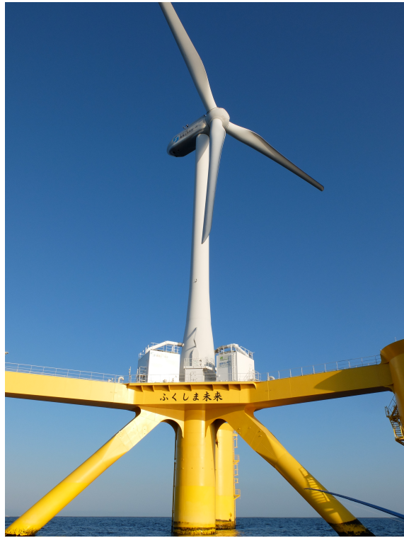
FIG. 2 Fukushima Future, the first floating turbine in the Fukushima offshore wind farm. Photo by author.
