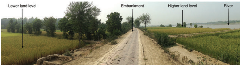
FIGURE 1.5. Embankment and raised banks due to siltation, 2014. Photo by author.
